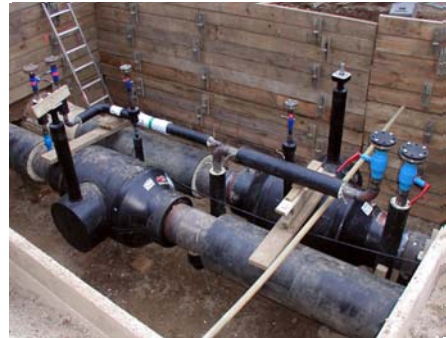
Ballostar ball valves pre-insulated, shown before and during the installation into a district heating network
