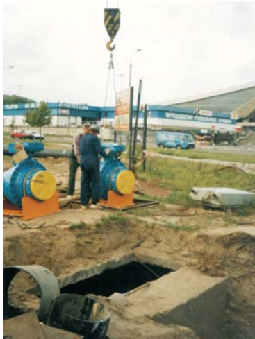
Installation of KLINGER Ballostar KHSVI in the North of Poland
